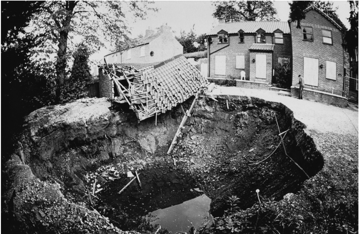
Fig. 1. The new sinkhole at Ure Bank Terrace, Ripon, looking northeast. The hole formed in April 1997, and measured 10 m across and 5.5 m deep. It was caused by collapse over a cave formed in gypsum of Permian age. Photograph by Tony Waltham.
