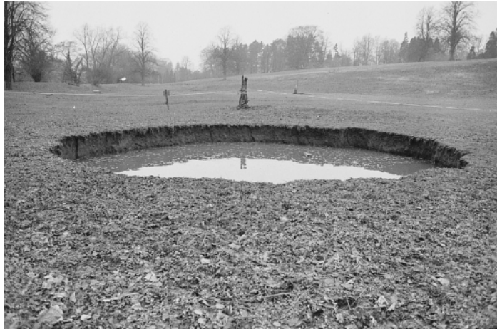
Fig. 5. Subsidence sinkhole that formed on 1 February 1982 at Sharow, near Ripon. The hole was 12 m in diameter and up to 9.7 m deep. Photograph by Tony Cooper.
